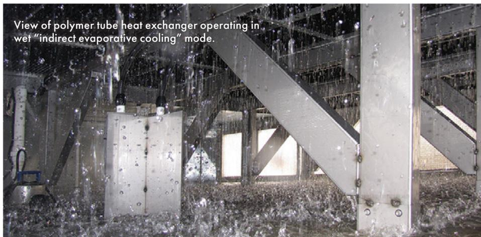
View of polymer tube heat exchanger operating in wet "indirect evaporative cooling" mode.
