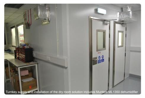
company in the past. After visiting site and reviewing customer needs, Munters recommended a turnkey solution for the supply and installation of a dry room with temperature and humidity control.
