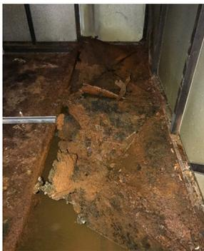
You might be surprised to learn that a unit in a bad condition (shown here) can still be brought back to life. Here you can see a Chilled water coil section that had a condense trap and drain problem. Over time, the water had leaked into the casework floor and had caused serious corrosion to the floor frame and panels. The coil was corroded so badly that it sagged in the middle, and was in danger of splitting completely. The
