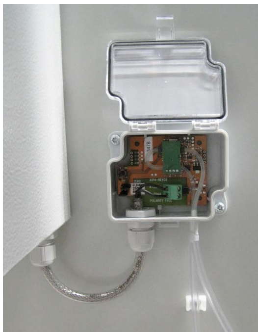
Figure 3.23 Connection for DPT (Process fan)
