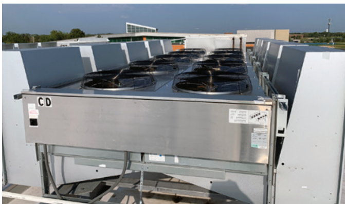
Patented modular "by-fan-bank" design concept has one CoVAP per condenser fan.
