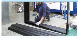
Start to mount the plastic waves: first the wave then the spacers.
