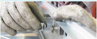
Place the oval plate over support frame and then start to screw the nuts.
