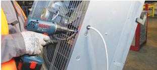
Fix the safety mesh guard to the housing with the screwdriver (ref.3/Assembling tools).
