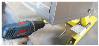
Fix the cover plate on each side by using q.ty 2 Ø6,3×19 screws (ref.2) with the screwdriver (ref.3/ Assembling tools).
