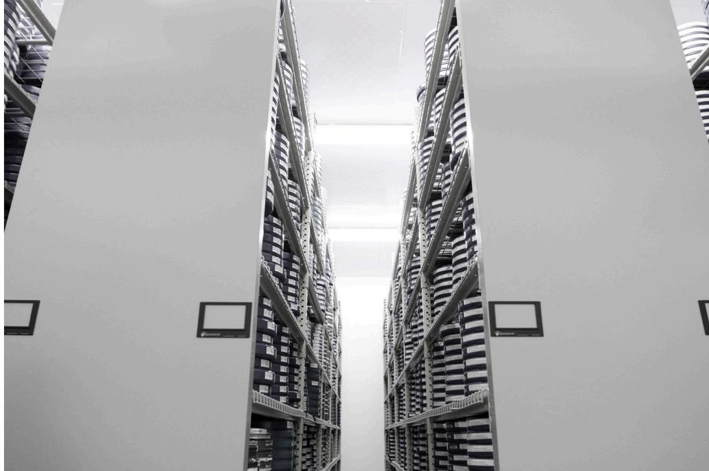
The HCD Plus provides a precise temperature of 45°F with a relative humidity of 25%, which was required to ensure the preservation of safety film reels for many years to come.
