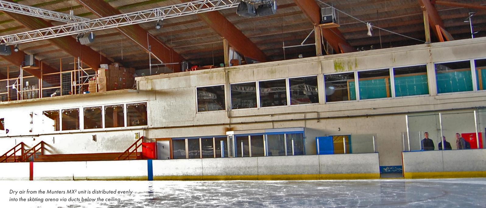
Dry air from the Munters MX<sup>2</sup> unit is distributed evenly into the skating arena via ducts below the ceiling.
