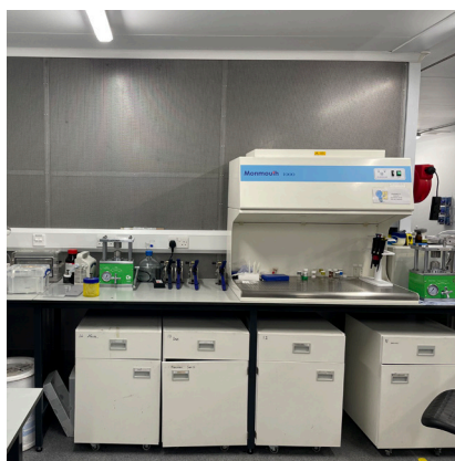
Air is supplied through the wall.
