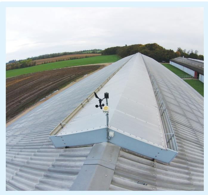
The weather station (installed on the ridge of the stable) provides information on wind speed, direction as well as precipitation. Controllers can be set to close curtains (or ridge vent) completely or gradually if it starts to rain or if the wind conditions change.
