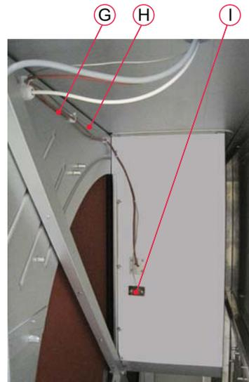
Abb 3.20 PT1000-Kabel (G), HTCO-Kabel (H), Rohr (I)
