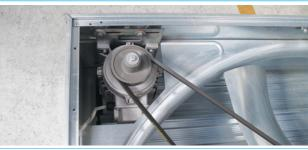
Turn the fan upside down and insert the electric cable into the proper hole placed on the side panel.
