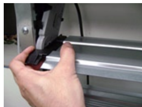
9. Replace the blade half blade and join it with the other half using the two bolts and nuts. Turn the magnet away from the override position back to the resting position (as in step 1)
