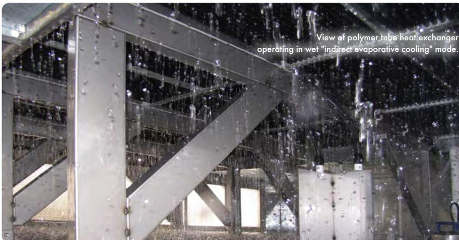
View of polymer tube heat exchanger operating in wet "indirect evaporative cooling" mode.
