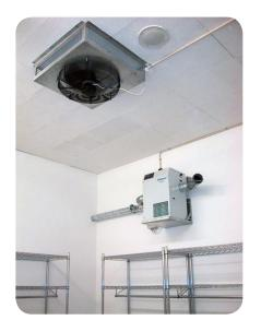
With Munters' drying solution, a desiccant wheel is used instead of wind. This promotes the release of dampness from the cloth to the air, from which the dehumidifier then removes the dampness.
