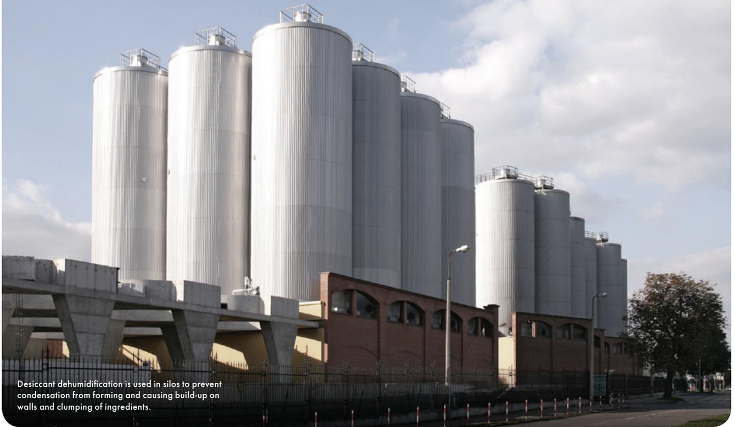
Desiccant dehumidification is used in silos to prevent condensation from forming and causing build-up on walls and clumping of ingredients.
