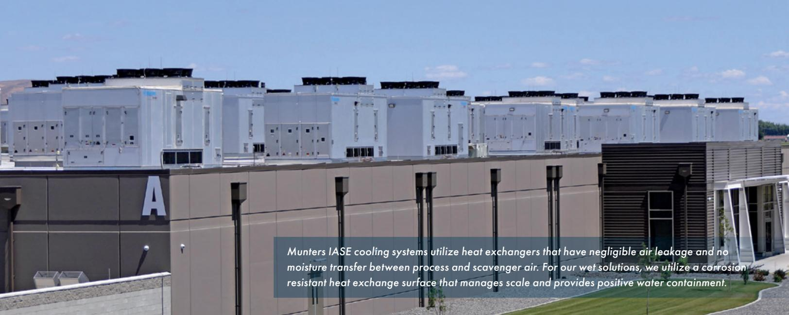
*Munters IASE cooling systems utilize heat exchangers that have negligible air leakage and no moisture transfer between process and scavenger air. For our wet solutions, we utilize a corrosion resistant heat exchange surface that manages scale and provides positive water containment.*
