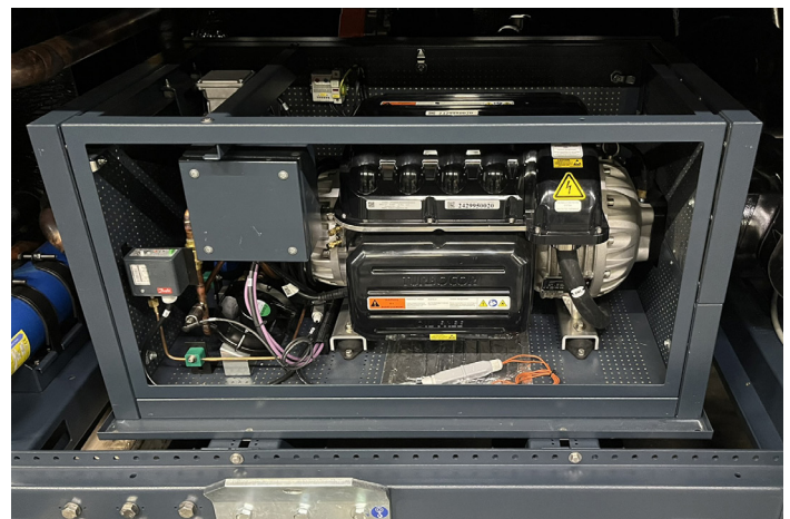
Insulated acoustic compressor enclosure example
