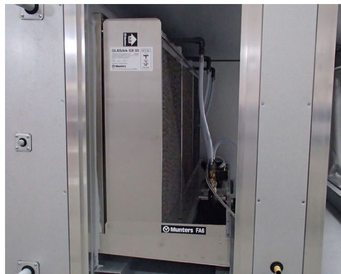
Example of an FA6 installation in a section of an airhandling unit
