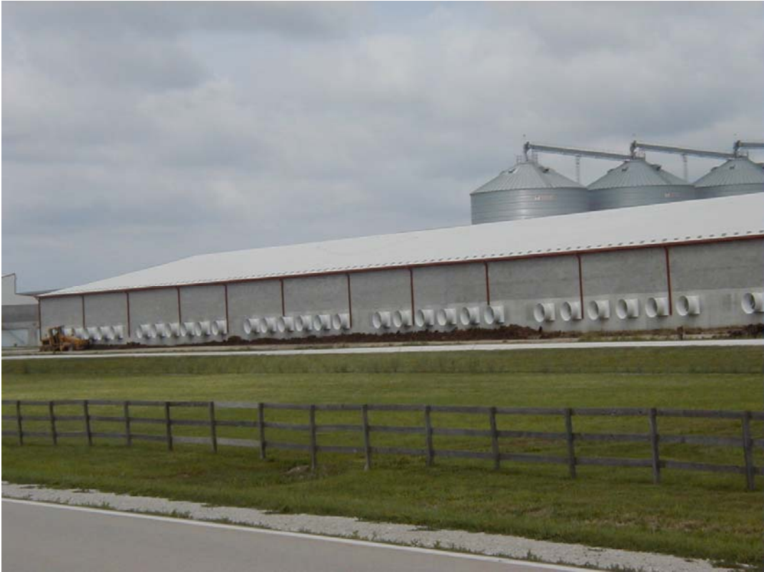
48" Advantage® fans in poultry layer building
