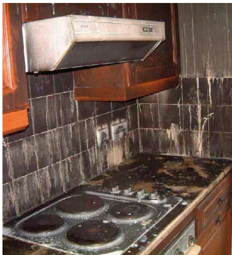
Smoke damaged kitchen.
