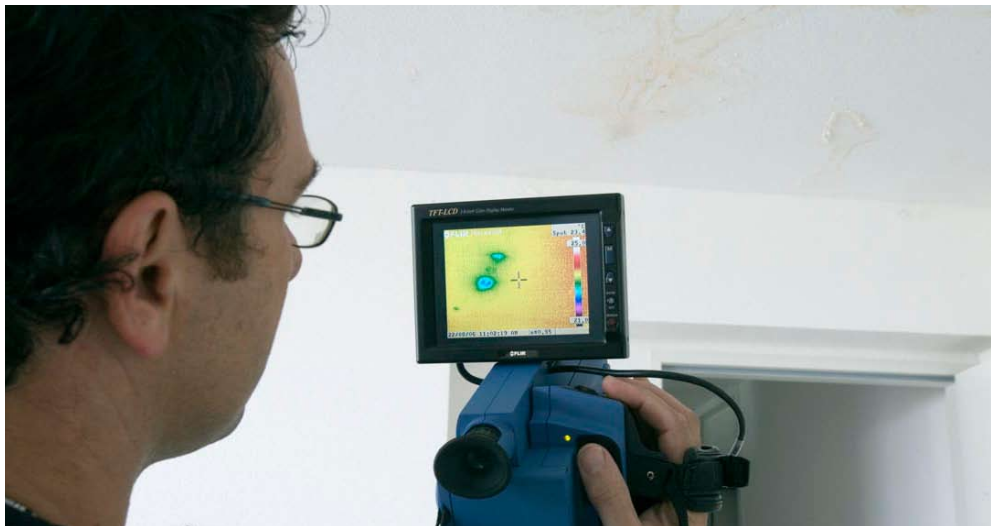
Using thermography to identify a pipe leak.
