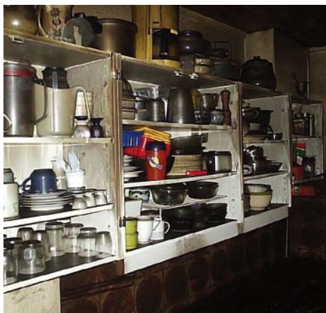
Kitchen and contents after fire before decontamination and refurbishment.
