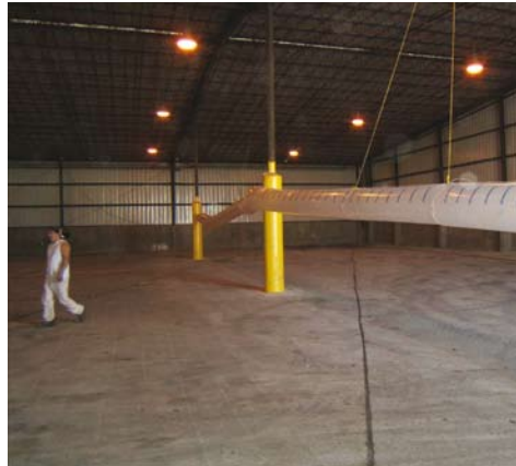
Drying progress will be monitored throughout the project.
