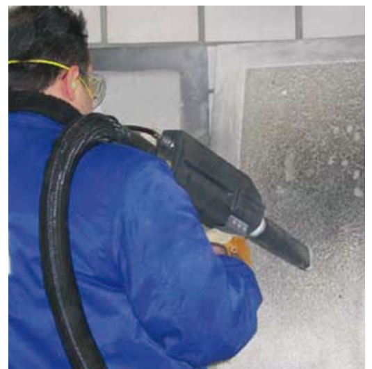
Cleaning with dry ice blasting machine.
