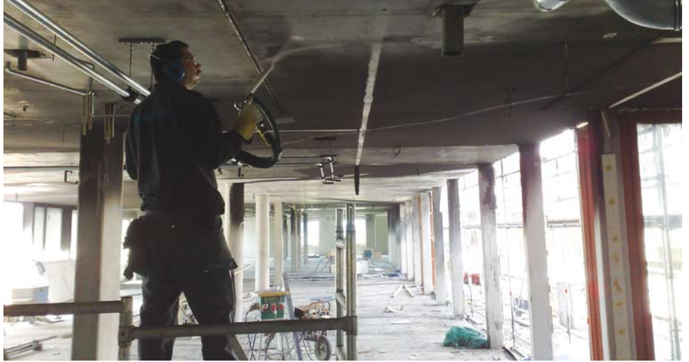
Dry ice blasting surfaces damaged by smoke.
