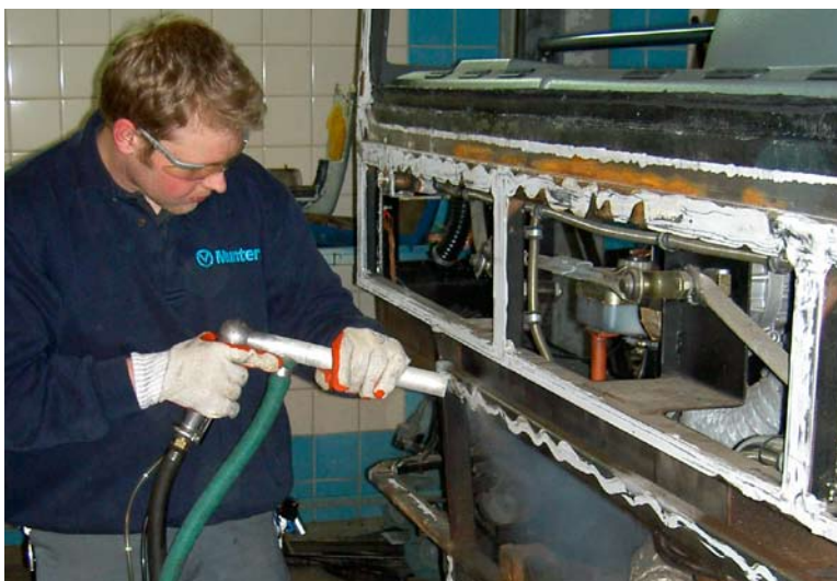
Dry ice blasting to reach hidden components.
