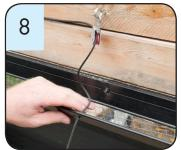
Pass the string through the hole in the curved louver then through the pulley, twords the direction of pulling force. Fix the string to the main pull cable or rod using clamp.
