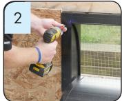
Fasten the left and right lateral side support using appropreite screws (2-inch or 5 cm). NOTES: Fastening points are marked on both supports. Screws and fittings are not included, Choose screws and fittings that are suited to the material in the wall and have sufficient holding power. If uncertain, contact Munters.
