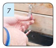
Install a small pulley at the top of the inlet. NOTES: Pulley or fitting are not included. Choose pulleys that are suited to the type of system or wall and have sufficient holding power. If uncertain, contact Munters.
