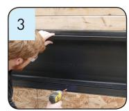
Fasten the bottom header profile using appropriate screw. NOTES: Fastening should be done in the center, on the marked line. Make sure the bottom header is straight (linear) when fastening.
