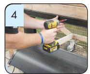
Push slightly up on the top header center, 0.25 inch or 0.6 cm. needed difference. Fasten the top header profile using appropriate screw. NOTES: Make sure the slight curvature of approximately 0.25 inch or 0.6 cm is achieved before fastening. Fastening should be done in the center, on the marked line.
