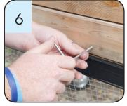
Fasten the (2) L-Screw hooks evenly spaced above header. Place 0.5 inch or 1.2 cm above the top header, opposite to the direction of pull.
