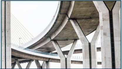
Dehumidification for Infrastructure
