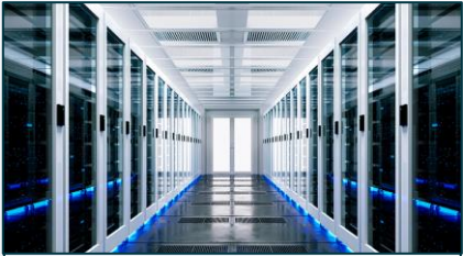
Cooling solutions for Data Centers
