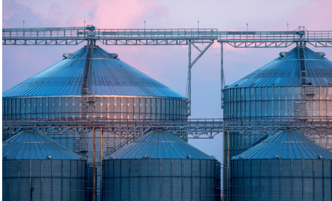
Dry air is fed into the blower used to convey ingredients from the truck to silos.
